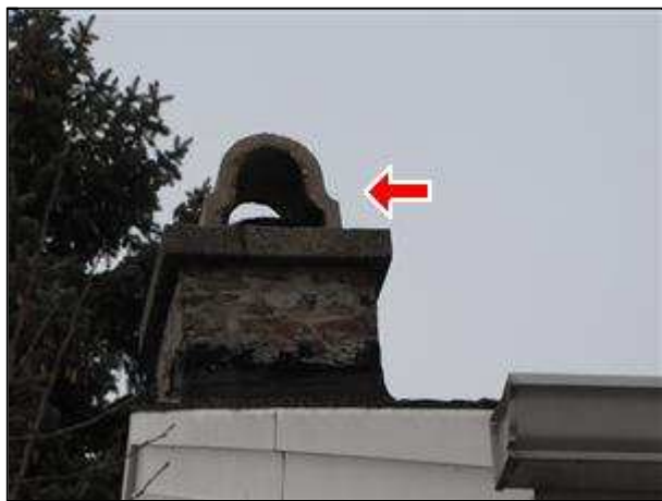
1.2 Item 1(Picture) Chimney has rain cap to prevent water intrusion.
