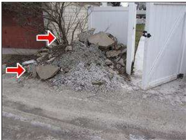
2.4 Item 1(Picture) Large concrete debris pile left in alley preventing gate from working properly.
